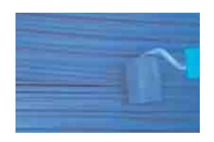
**STEP 4** Before applying to the roof, make sure that the "ReadySolar" is the right way up. Small holes are located along the length of the absorbers to allow rain water to be drained. Make sure that the holes are not blocked especially on a flat roof. <u>Do not</u> use screws in these holes to fix the absorbers.
